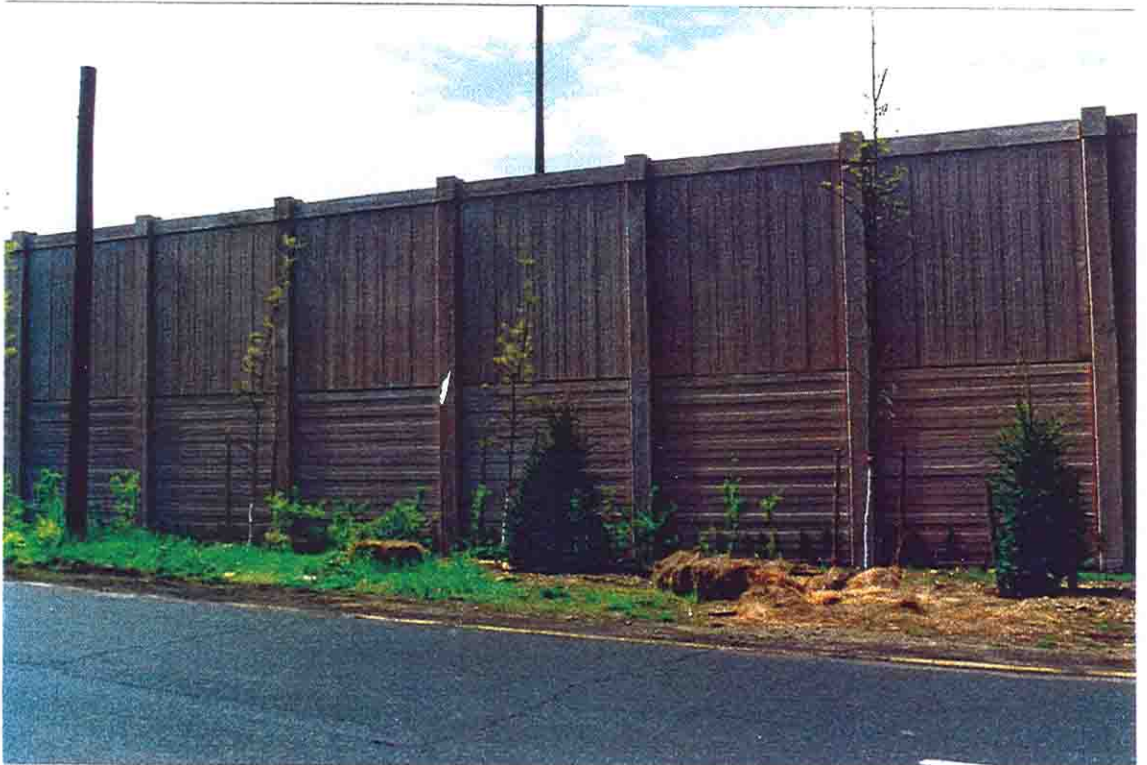
Below-- NYSDOT Post & Panel Noise Wall (view of residential side) SOBE-Route 495 Interchange, Plainview New York
