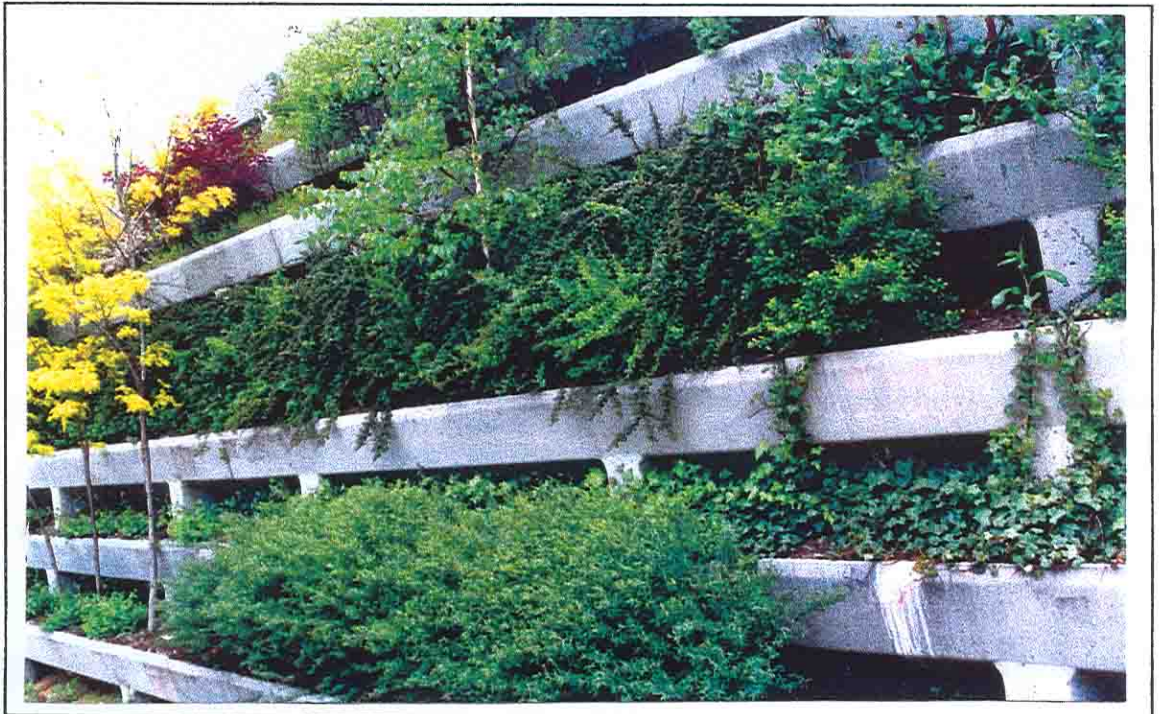
Picture 2 (South side)
