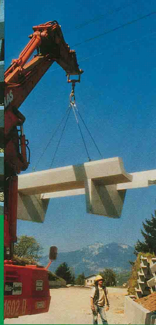
Curvalinear Retaining / Sound Wall
