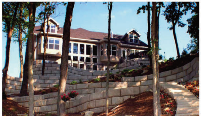
RESIDENTIAL RETAINING WALL
