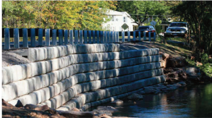
STONE RD., LOCKPORT - RETAINING WALL APPLICATION
