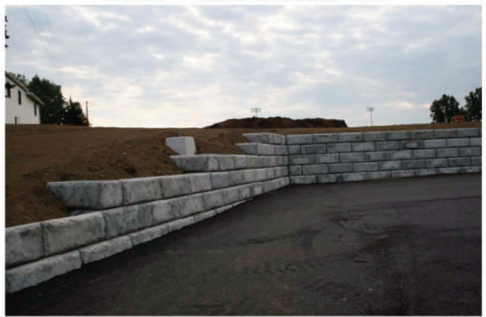
WEST SENECA CSD BUS GARAGE PARKING LOT
