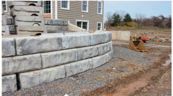
CURVED RETAINING WALL
