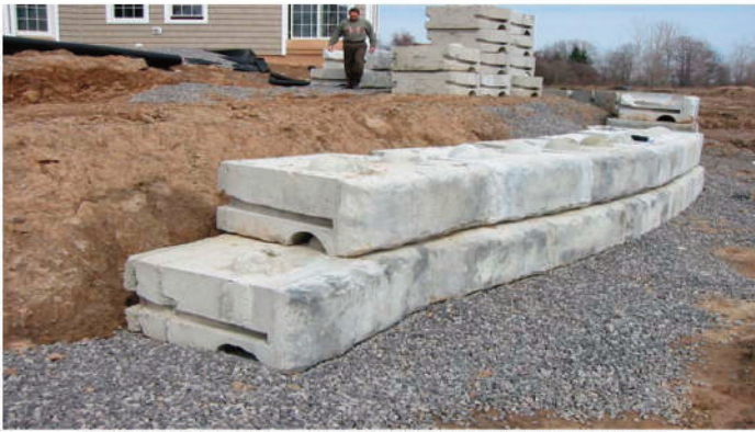
RETAINING WALL INSTALLATION IN PROGRESS
