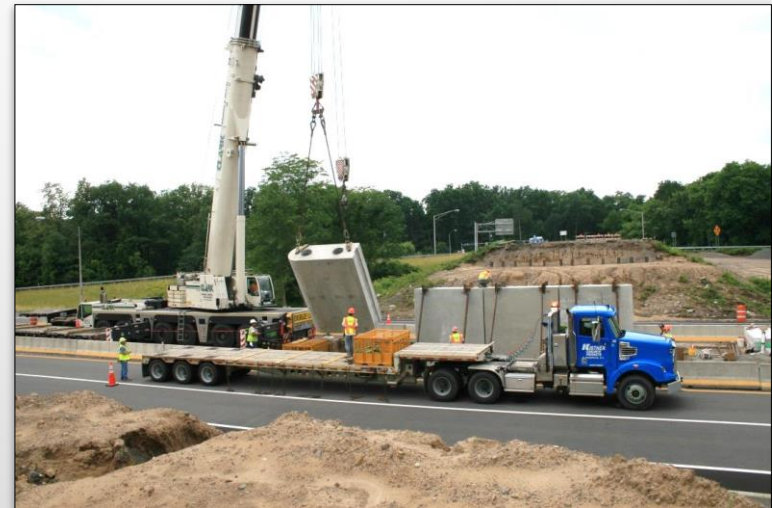
PRECAST BRIDGE PIERS
