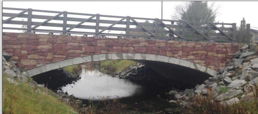
36' SPAN POTSDAM, NY
