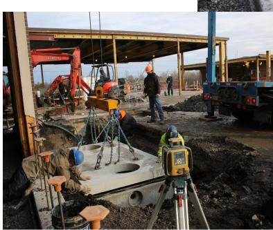
Tanks & Covers are unloaded & sealed using OSHA approved & engineer rated Lifting equipment for all product handling & setting.
