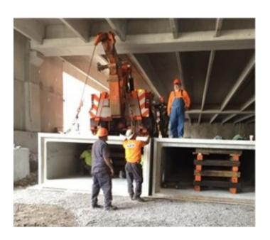
Low headroom made for a tricky installation of the large Precast Sections. A clever handling process was developed to accommodate the site conditions for a successful install.
