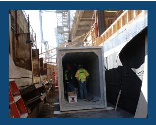
The Stormwater system needed to be placed between a lagging wall holding up the street and the buildings foundation wall. This left less than two feet of clearance on either side.
