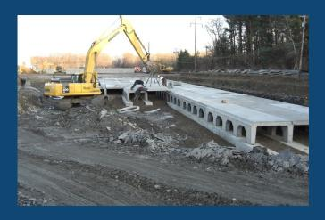
Tunnel style systems are also available for detention and infiltration applications. The picture to the left shows a tunnel style detention system at a Goya plant in Angola, NY.
