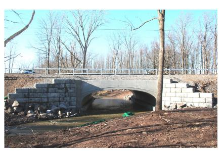
Sections of 28'-0" Span 22 Tons Arched Culvert sections, per AASH-TO HL-93 Loading. Detached precast headwalls.
